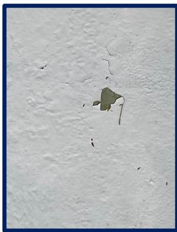
Peeling and flaking plaster on pool surface floor and walls.
