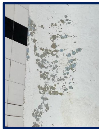
Peeling and flaking plaster on pool surface floor and walls.
