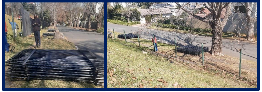
NEW PALISADE FENCE ON STURDEE AVE ( GDE FINANCED)
